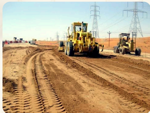
ROAD GRADING & EARTHWORKS
